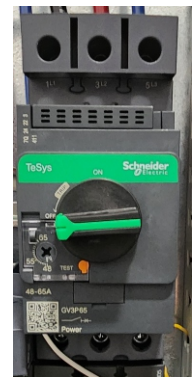
Heater Overload Tripped (OFF)
