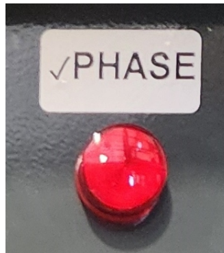
3. Phase Monitor ALARM Light (ON = OUT OF PHASE)
